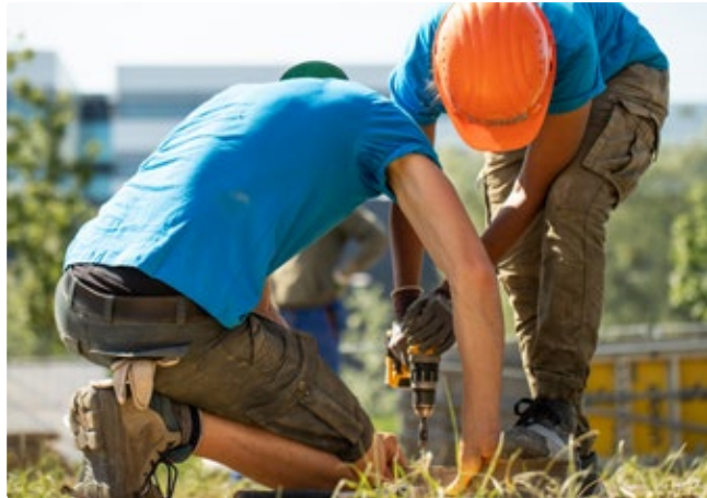
Construction of the formwork
