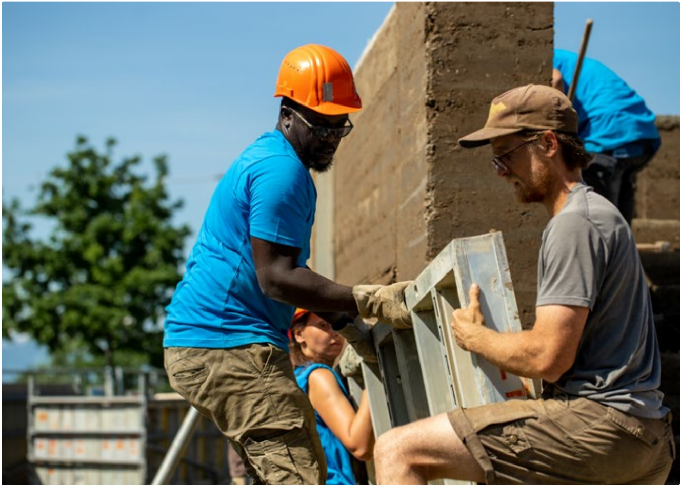
Formwork disassembly
