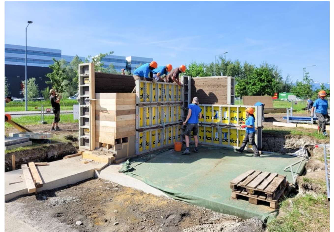
Formwork disassembly
