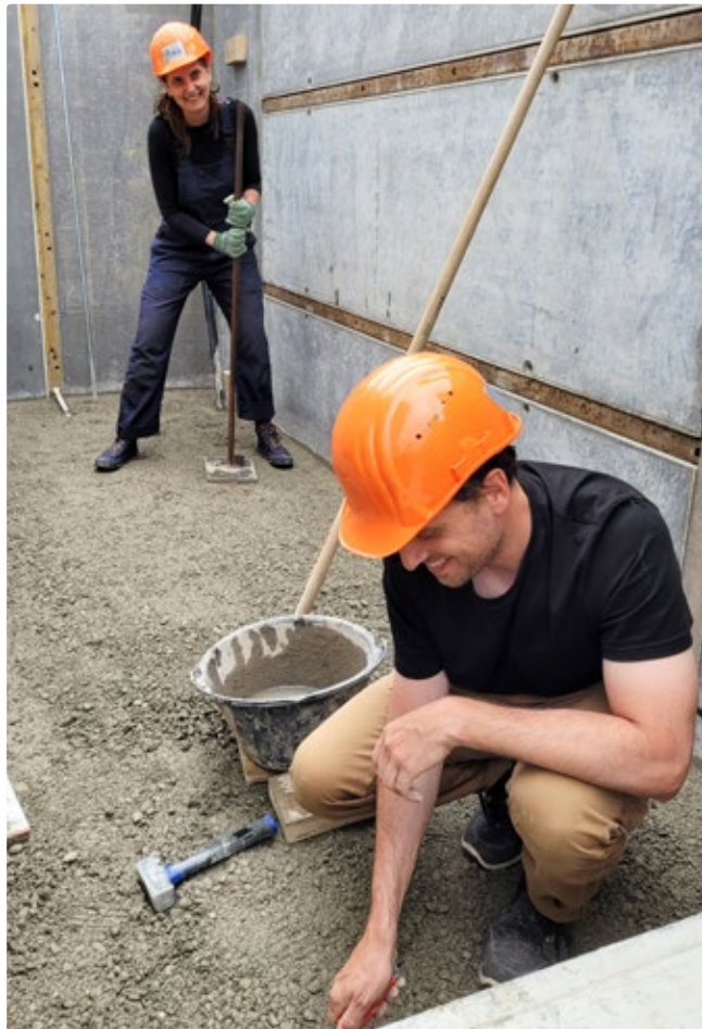
Preparation of the base of the wall
