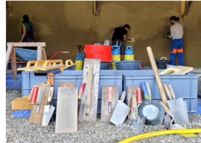
Tools for plastering
