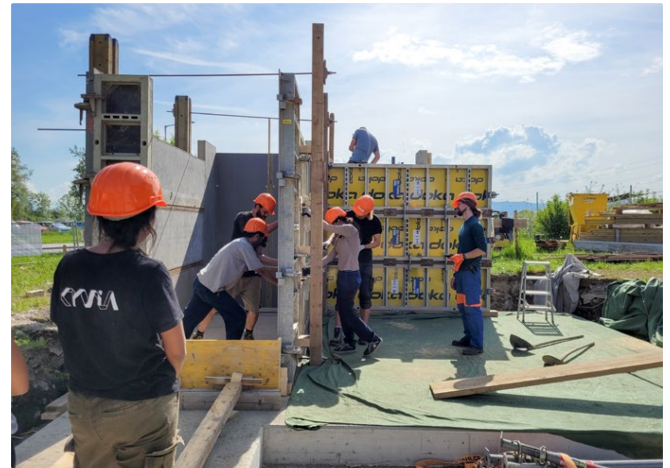
Preparation of the formwork
