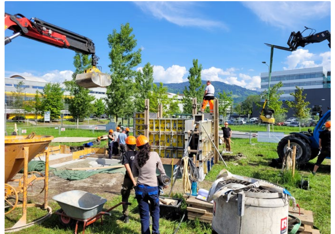
Overview of the construction site
