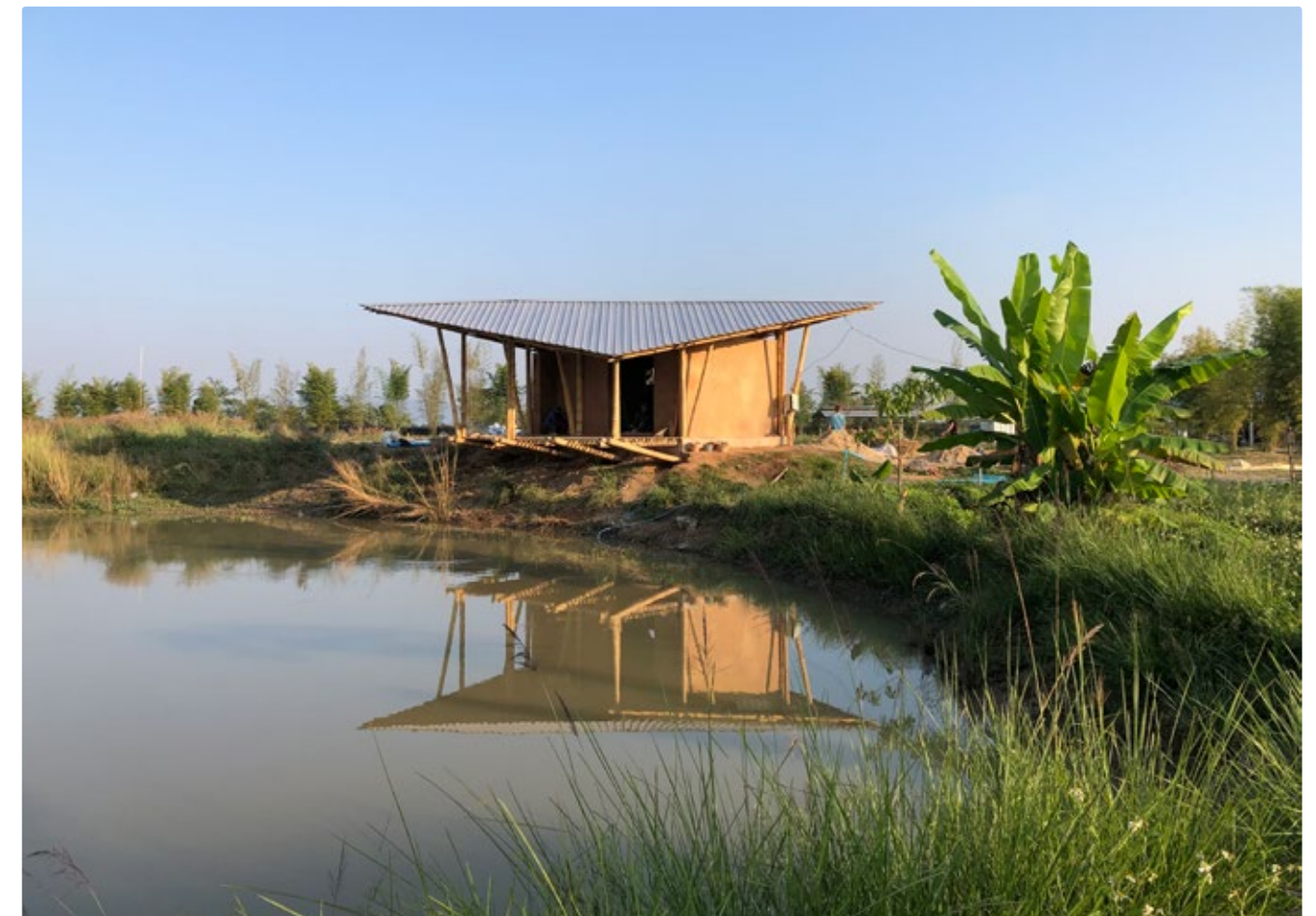
View of the finished guest house
