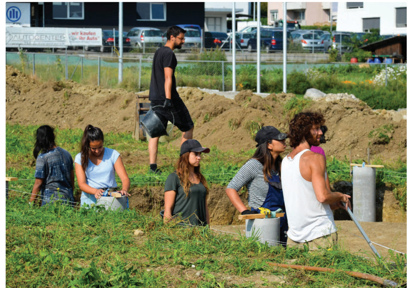
Placement of concrete pipes as foundation for the timber roof construction
