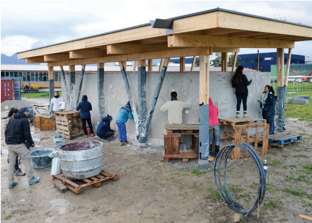
Applying lime plaster on the outside wall
