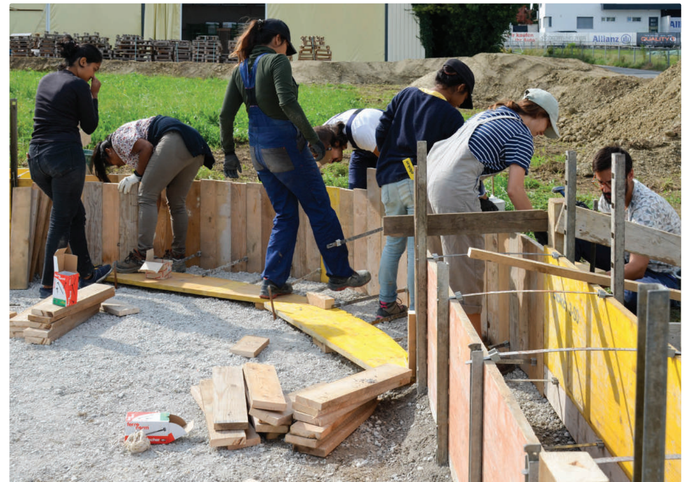
Building the formwork for the foundation wall
