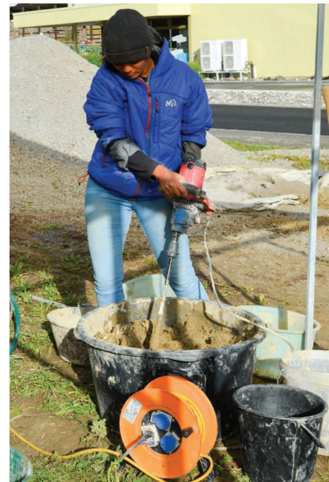
Preparation of the earth mortar
