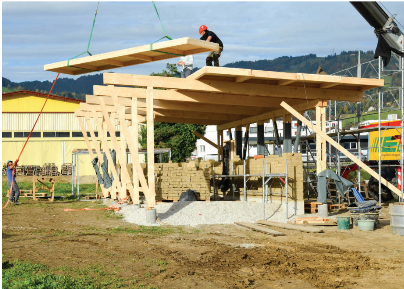
Assembly of the frame on the construction site
