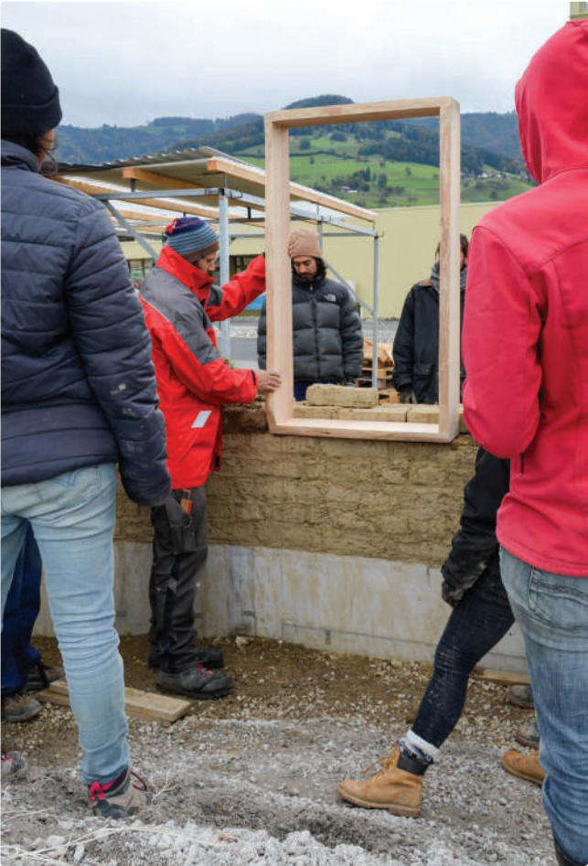
Placing the table frame inside the adobe wall
