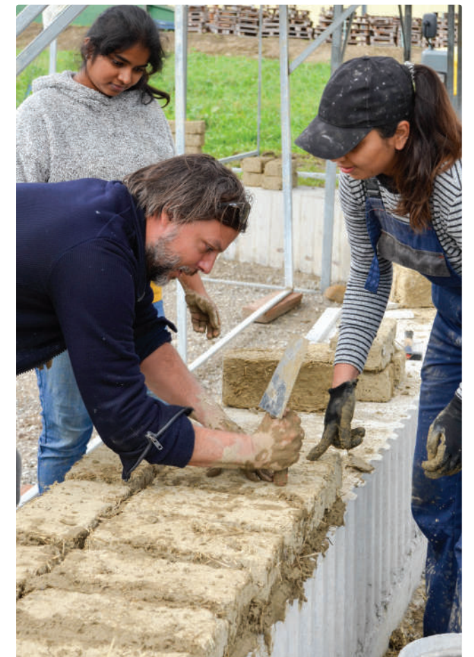
Laying adobe bricks under the supervision of Jan Glasmeier
