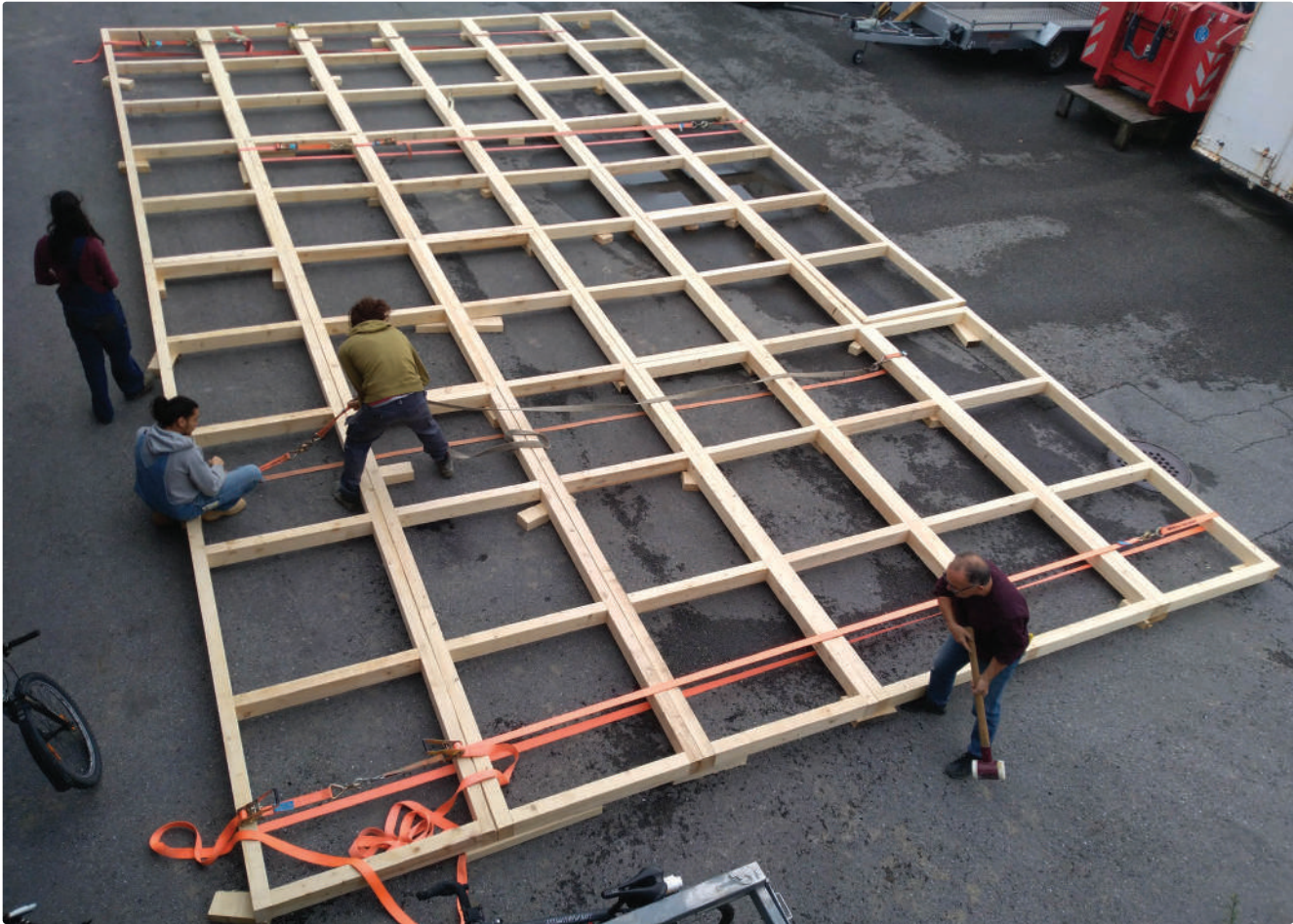
Wooden frame of the roof
