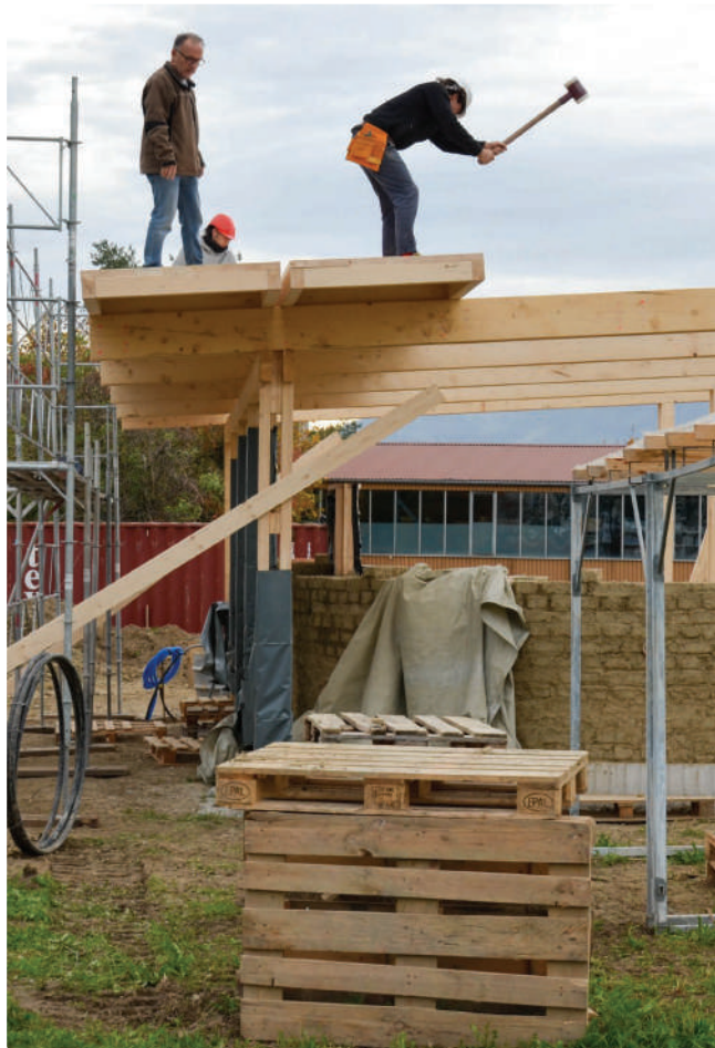
Assembly of the frame on the construction site
