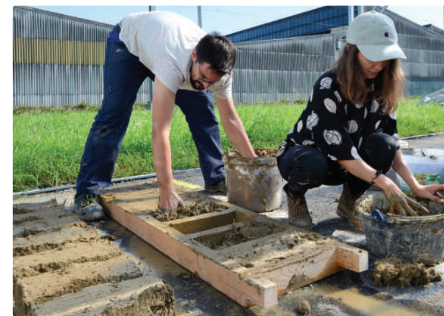
Formwork made with recycled wood
