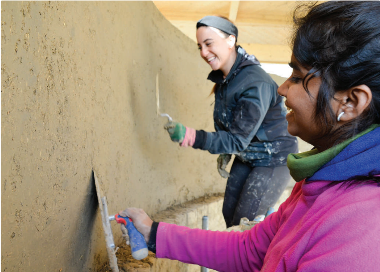
Clay plaster on the inside wall
