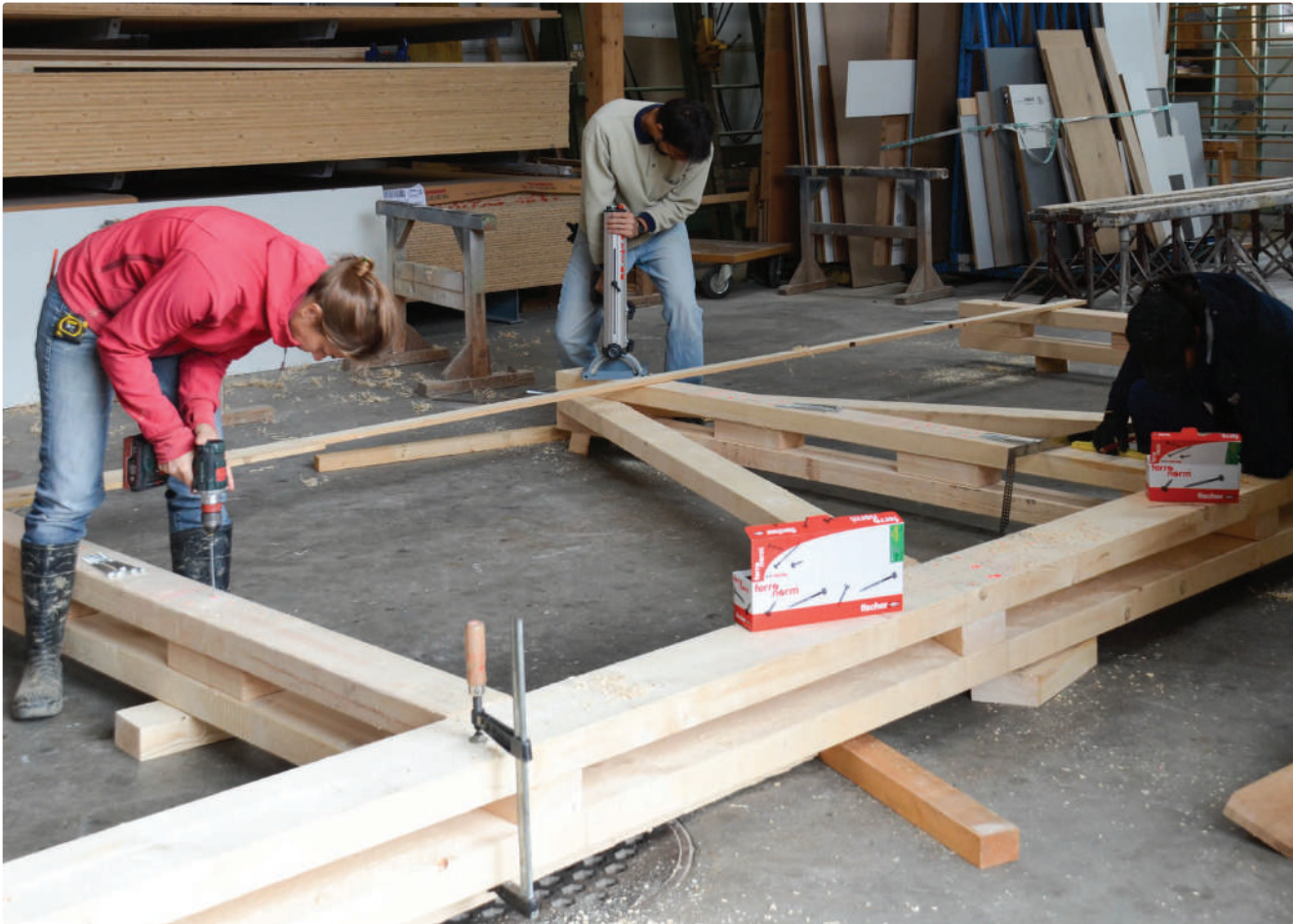
Preparation and assembly of the columns and beams
