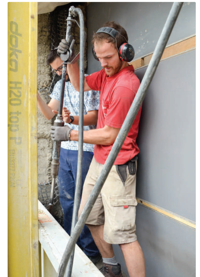
Construction of a rammed earth wall
