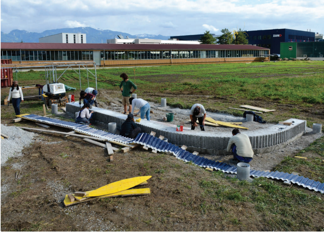
Dismantling of the formwork of the foundation wall
