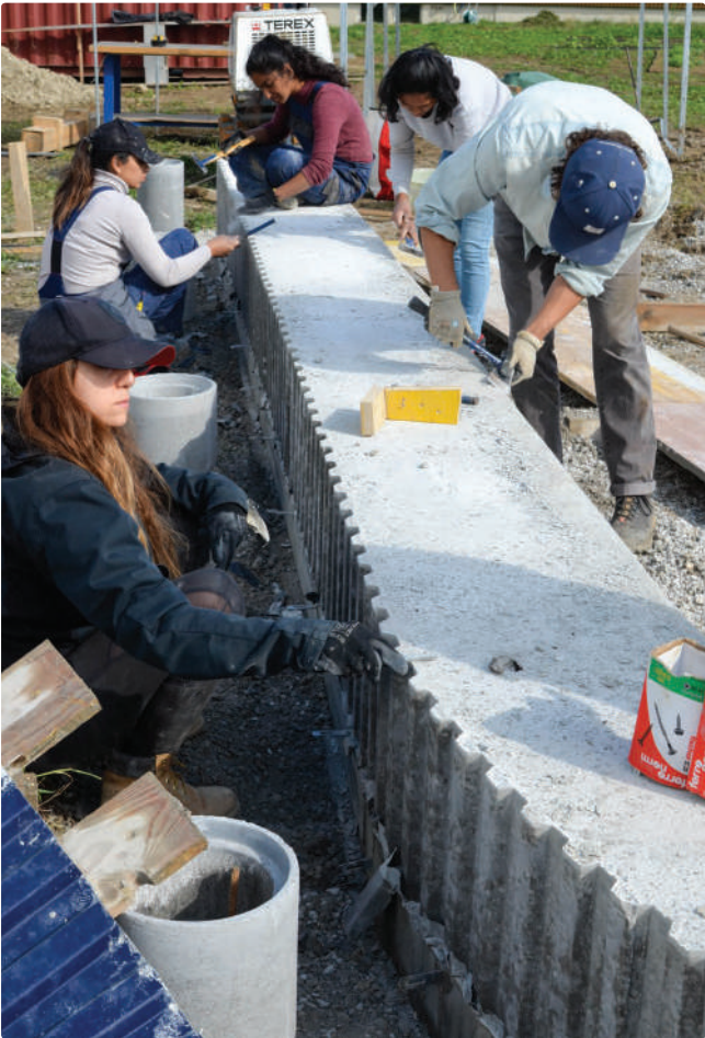
Detail of the foundation
