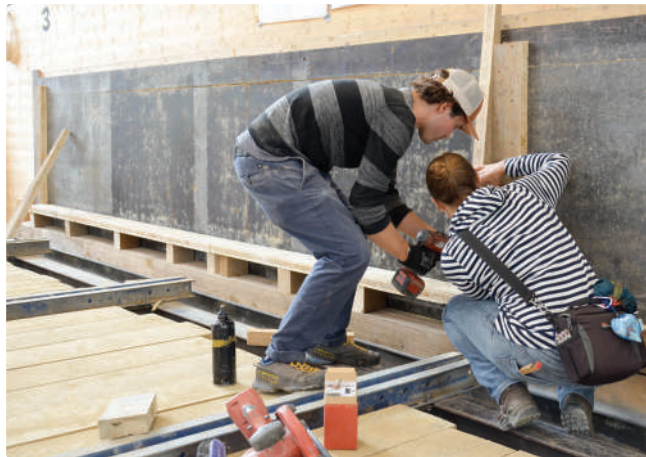
Construction of the formwork
