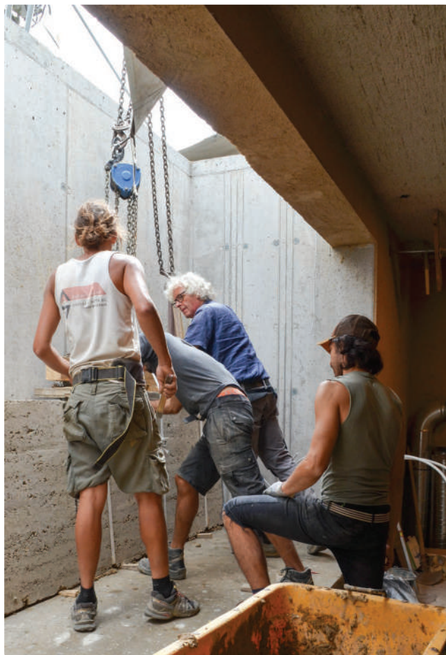
Placement of the prefabricated walls in the basement
