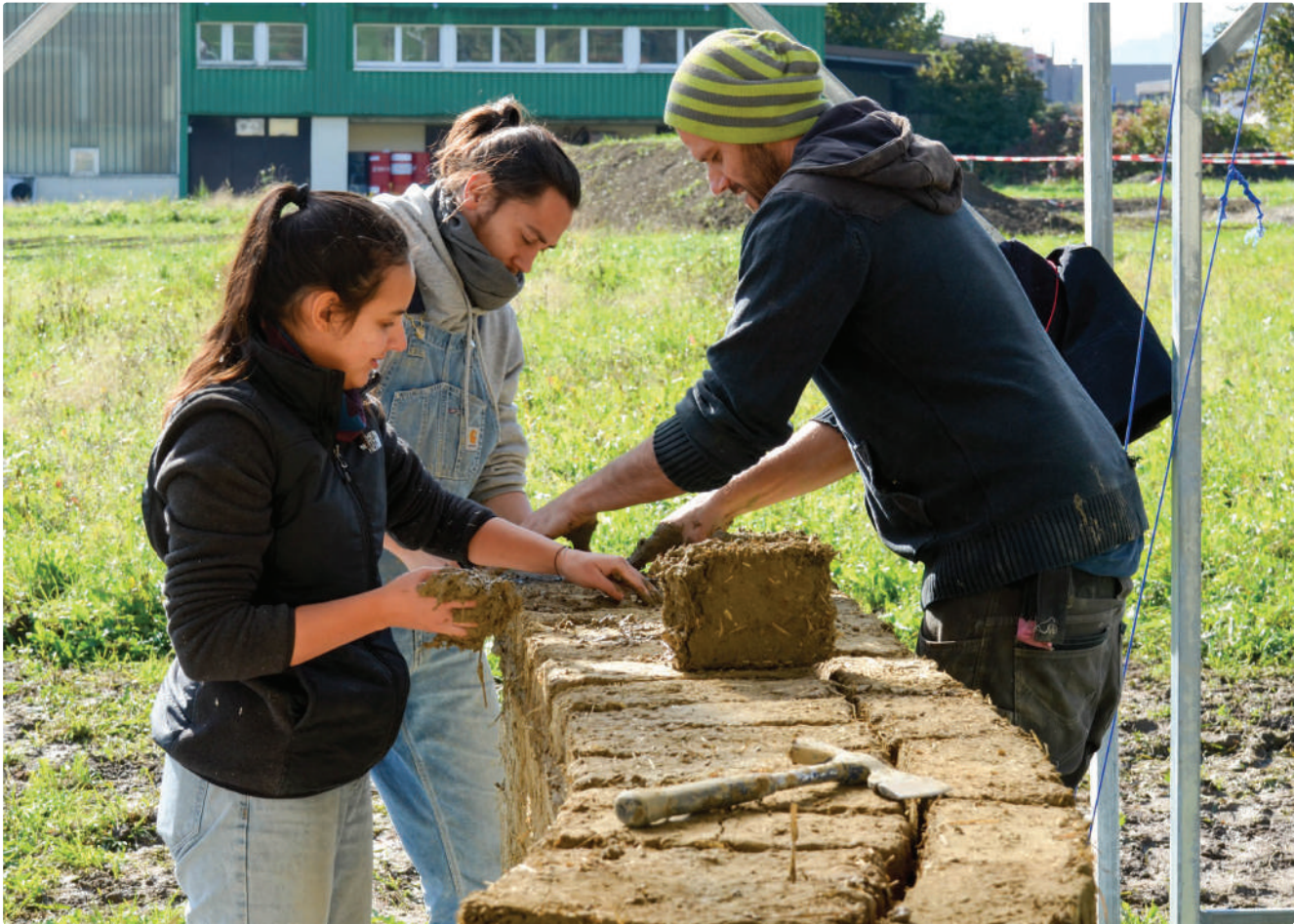
Adobe wall construction under the supervision of Dominik Abbrederis
