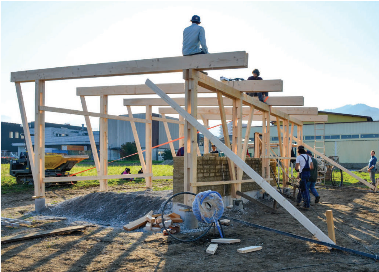
Assembly of columns and beams on the construction site
