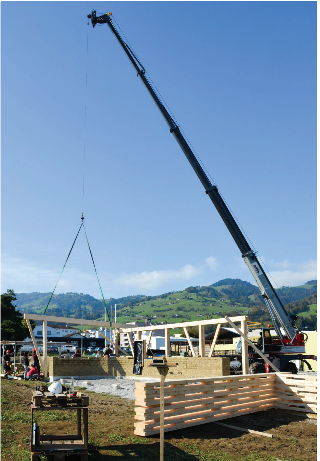
Assembly of the structural parts on the construction site with the help of a small crane
