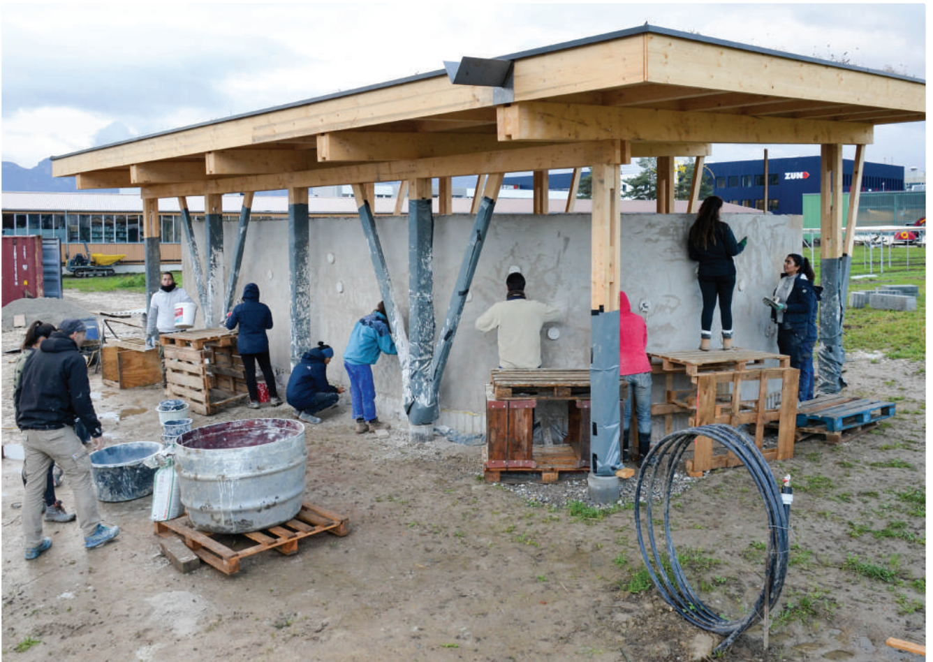
Applying lime plaster on the outside wall
