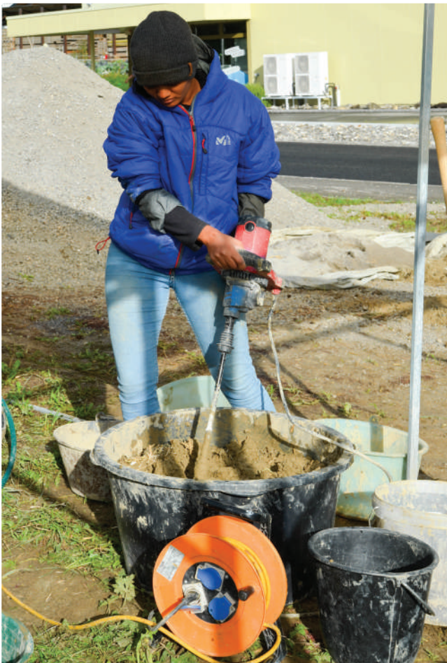
Preparation of the earth mortar
