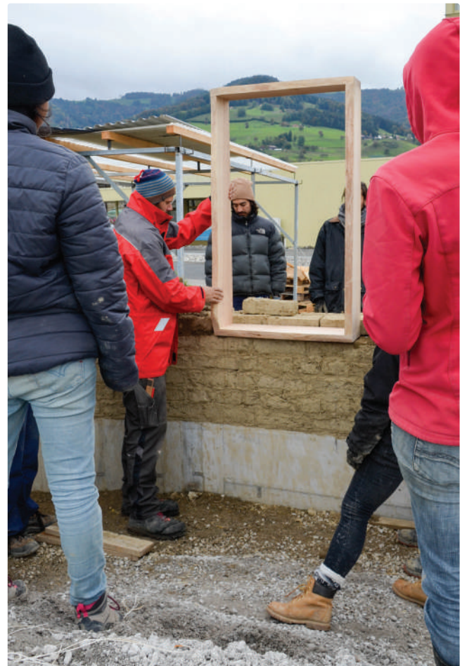
Placing the table frame inside the adobe wall
