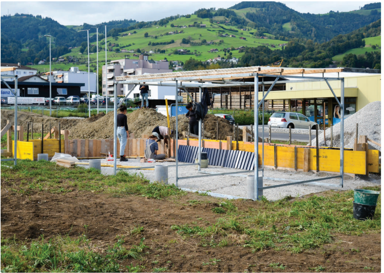
View of the formwork and concrete pipes
