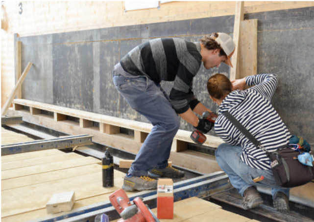
Construction of the formwork
