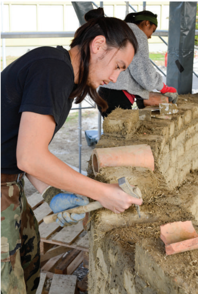
Placing recycled clay pipes on the back of the wall
