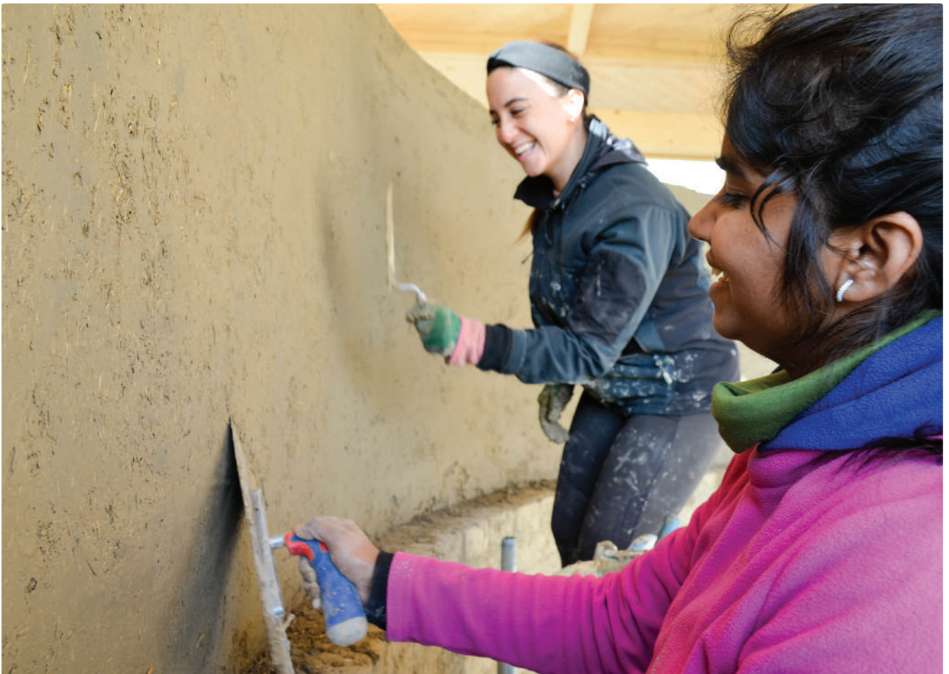
Clay plaster on the inside wall
