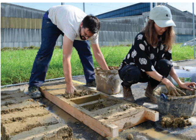
Formwork made with recycled wood
