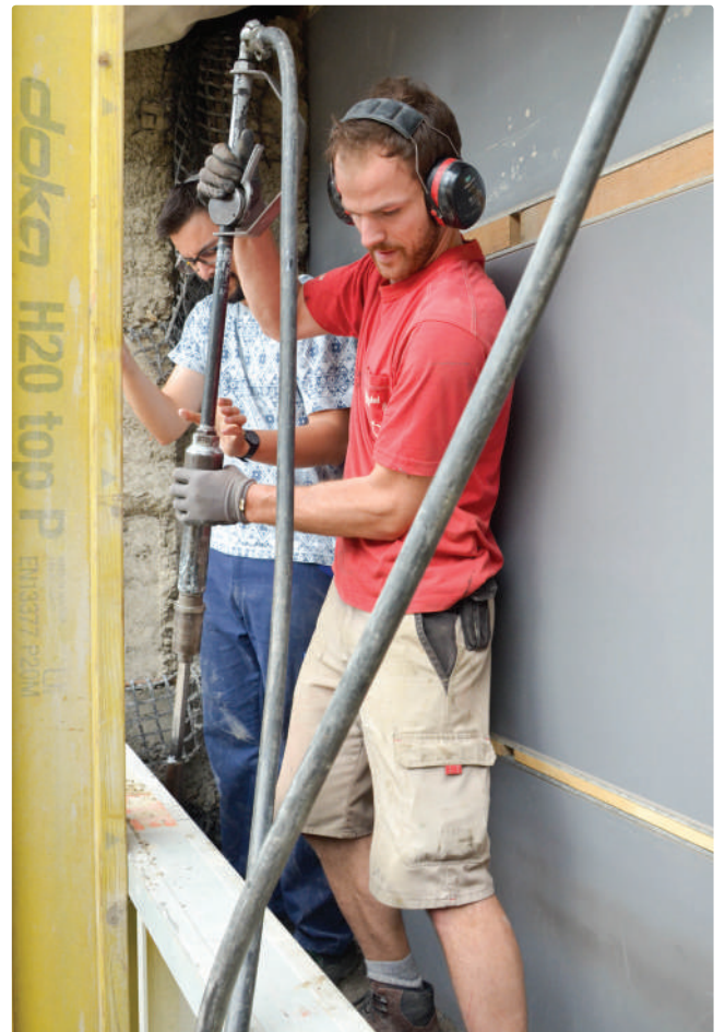
Construction of a rammed earth wall
