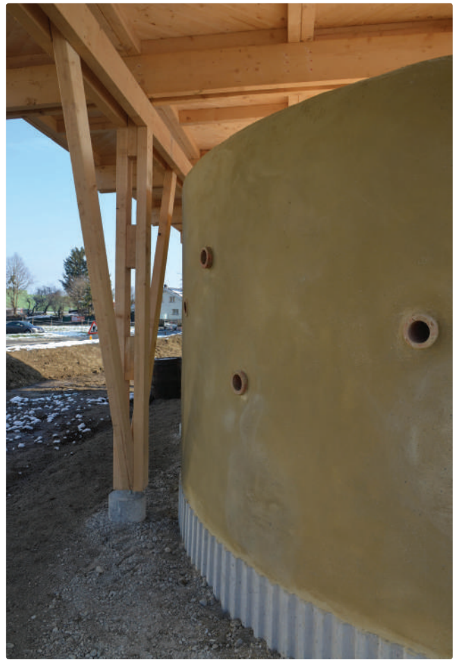
View of the back facade with recycled clay pipes used as decorative elements
