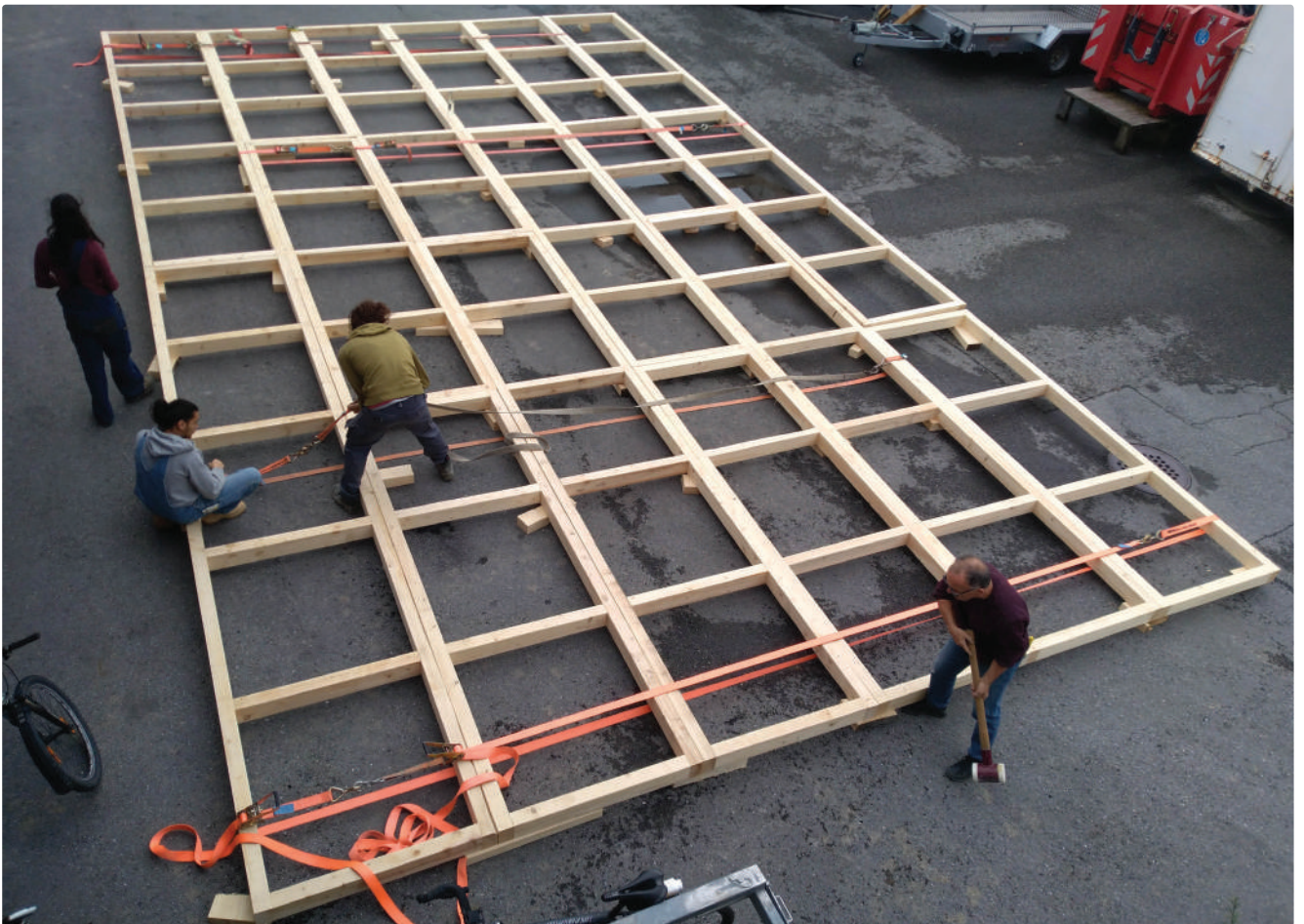
Wooden frame of the roof
