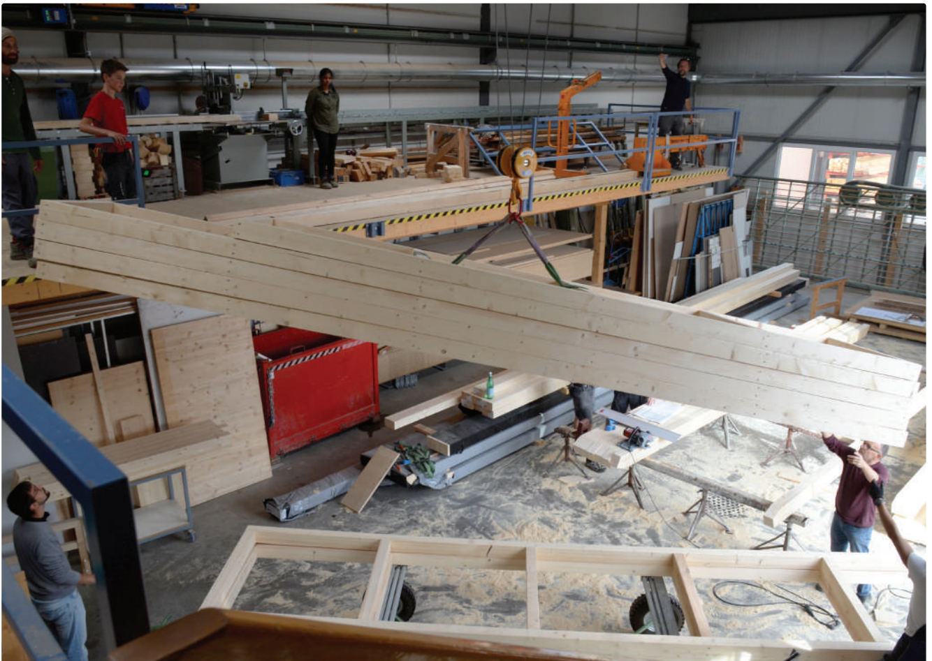
Preassembly and transport of the elements to the construction site
