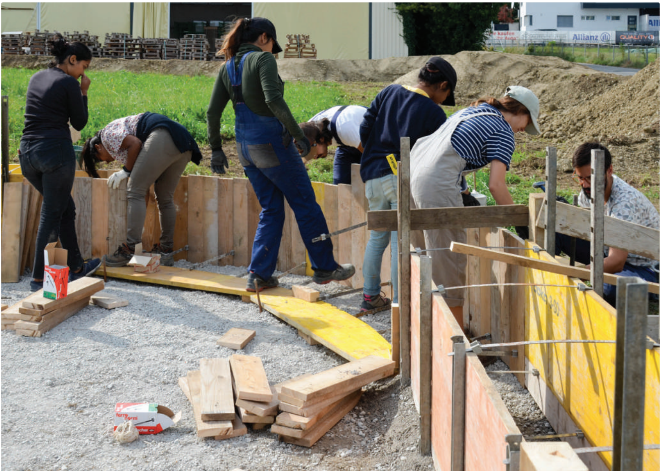
Building the formwork for the foundation wall
